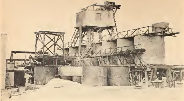
Semicommercial pilot nitrate recovery plant at Oficina Cecilia, Chile, built about 1922, with a capacity of 40 tons of ore per day. Here the pioneering of the new process was carried out.
